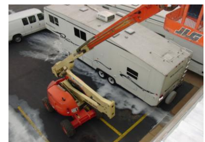
Pictured right, recreational vehicle having its exterior coated with Super Therm® and topcoated with Enamo Grip.
