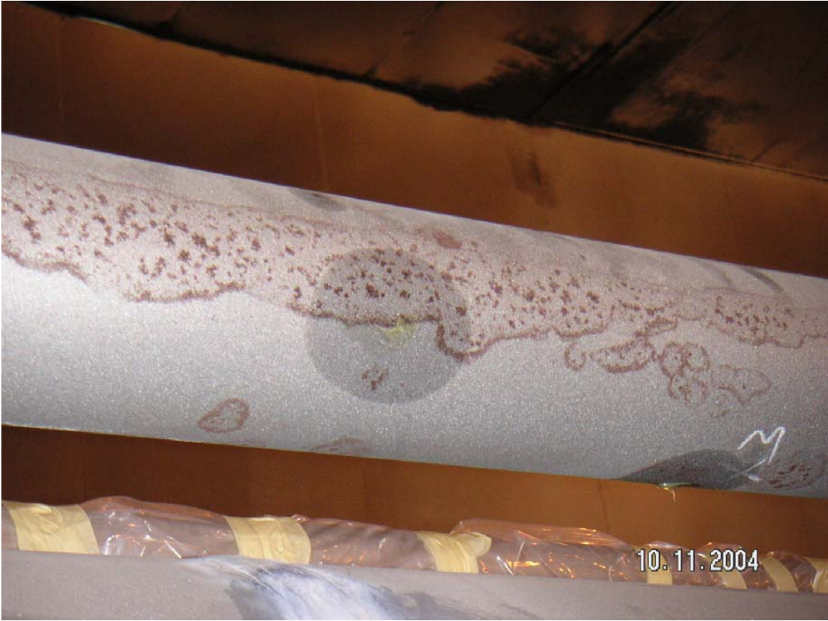
4. First batch sand blasted
